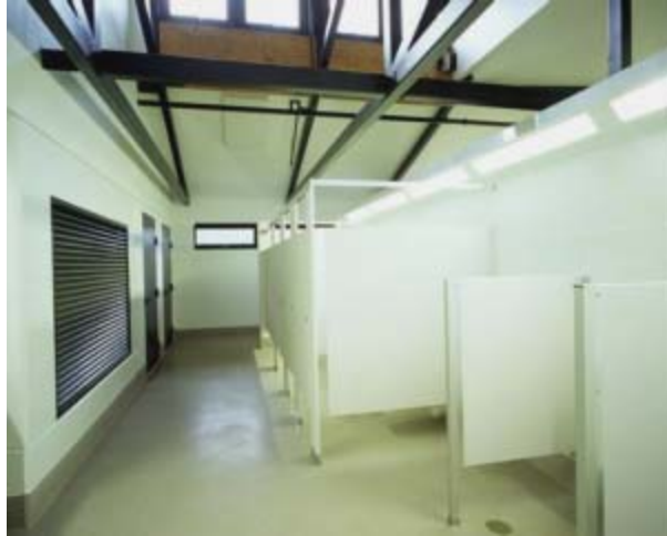
Figure 4-8 Lighting in Comfort Station
