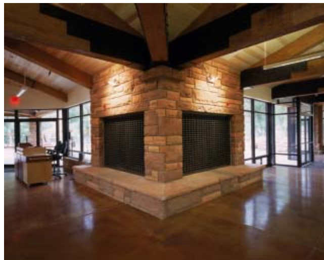
Figure 4-17 Interior view of a cooltower showing operable shutters that allow cool air to enter the building through the bottom louvers
