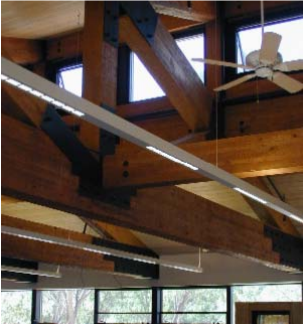
Figure 4-7 T-8 space lighting (note the dark ceilings and minimal down lighting)
