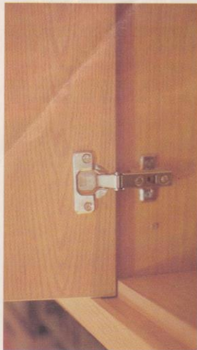
Above: The door hinge and frame on the bottom part of the unit
