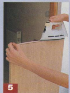
5 Applying edge banding on manufactured board
