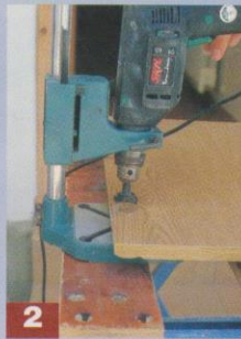
2 Drilling doors to accept hinges
